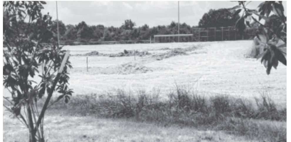
The irrigation system at Milltown Park receives upgrades
