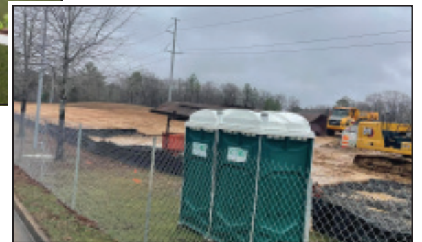
Construction was underway earlier this year at the Rankin site.
