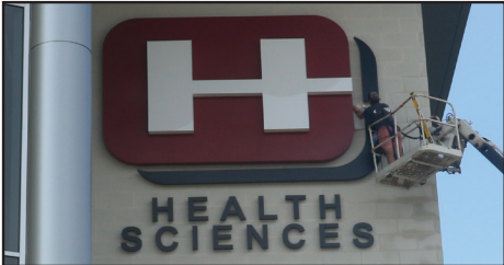
The Hinds Community College "H" was installed on the school's new Health Sciences Complex using a crane, just in time for the start of classes on August 10.
